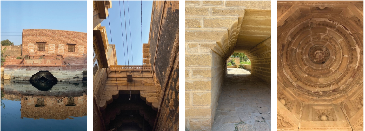
Figure 17 Simplified form of corbeling seen in the roofs and as supports in the region
