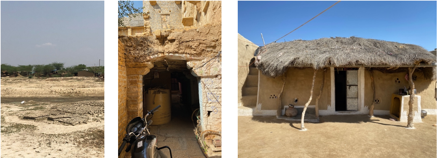
Figure 4 Making and use of mud in the various types of buildings in the region
