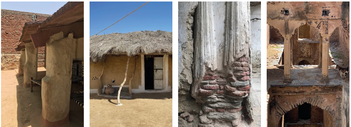
Figure 12 Types of columns seen in the region
