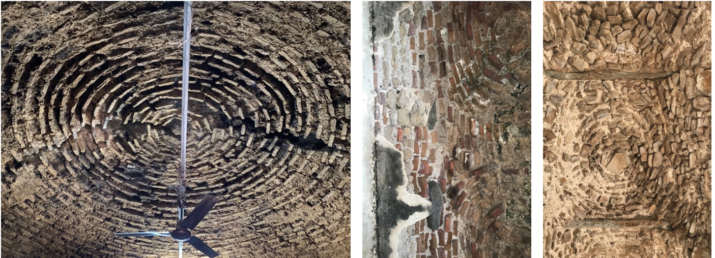
Figure 18 Multiple geometries and materials used in the dolas roofs
