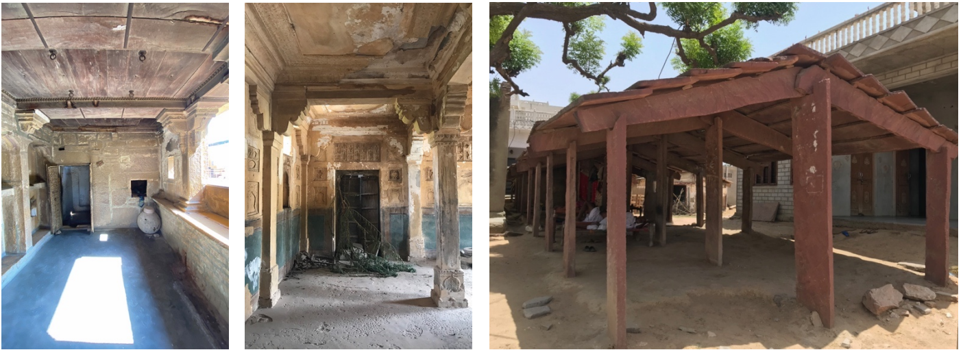
Figure 14 Spatial variation in the use of trabeated construction seen in the region
