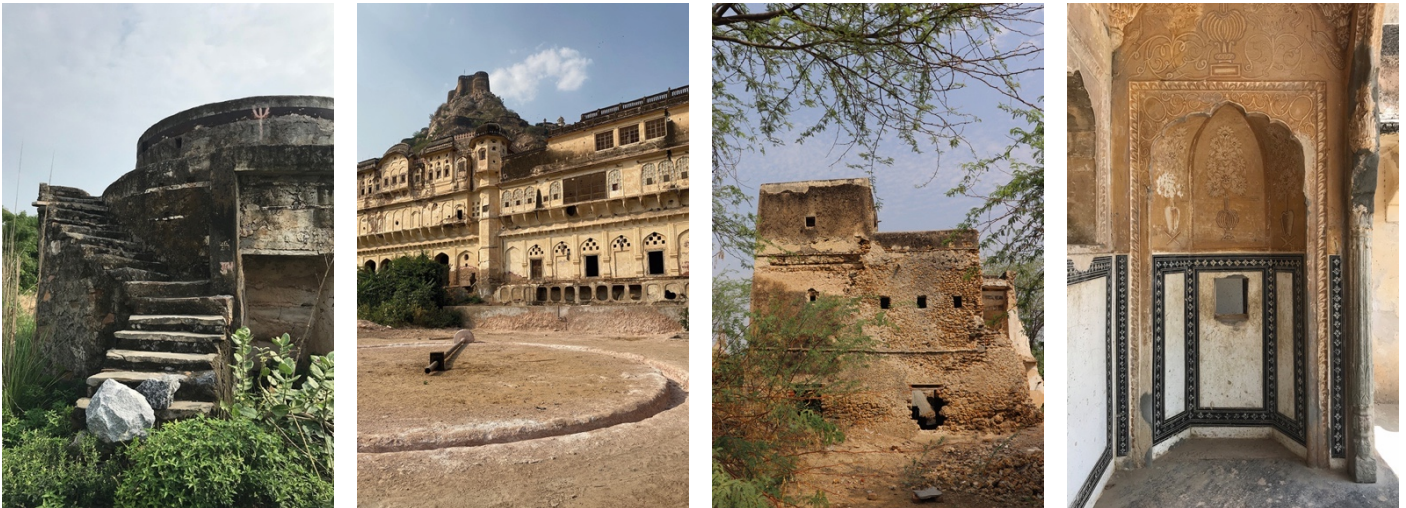
Figure 11 Infrastructure for lime plaster preparation processes and uses
