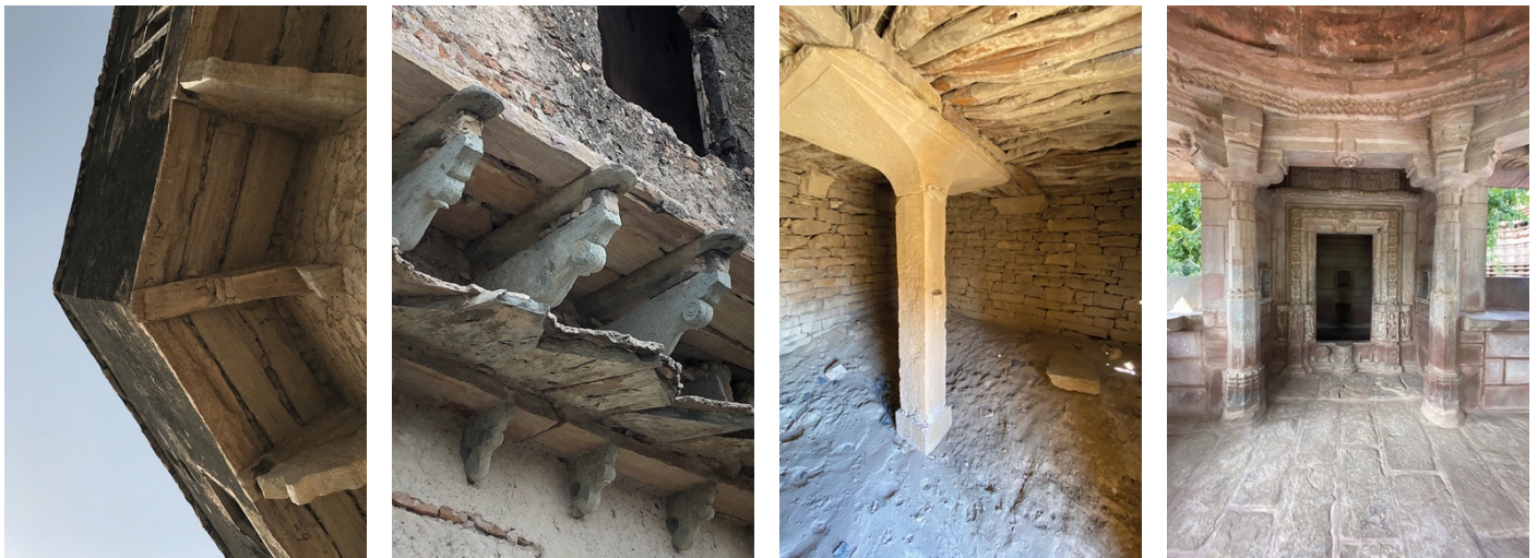
Figure 13 Multiple kinds and uses of brackets
