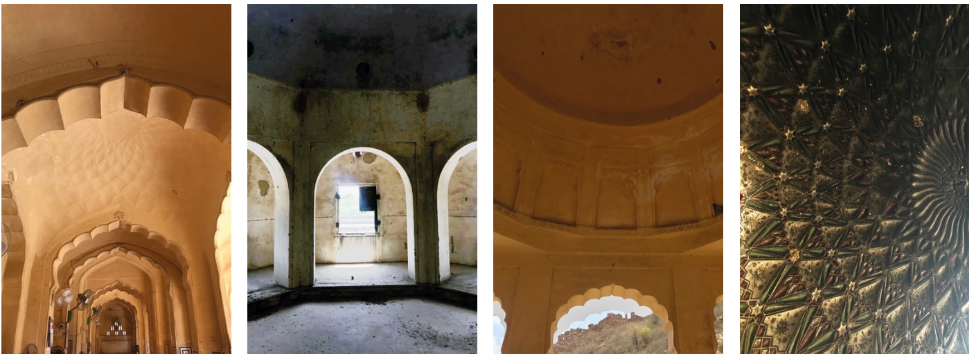
Figure 23 Squinches, Muqarnas and pendentives are used to support the masonry domes and half domes
