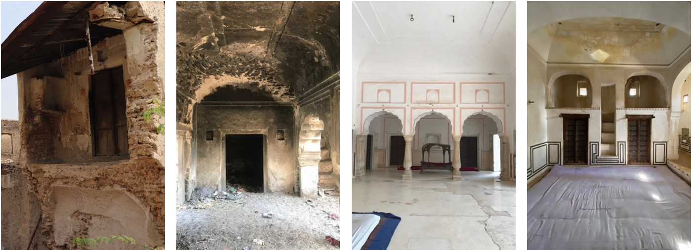
Figure 19 Make and finishes of the various types of Dola roofs
