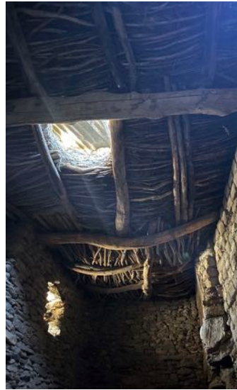
Figure 56 Opening in the terrace floor to transfer hay to the floor below
