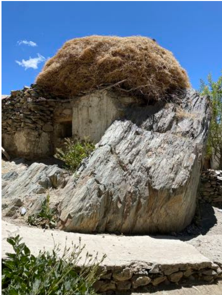
Figure 41 & 42 Construction of structures have complemented and used the natural terrain. Big immovable boulders are accommodated within the structures as seen in Karsha and Padum
