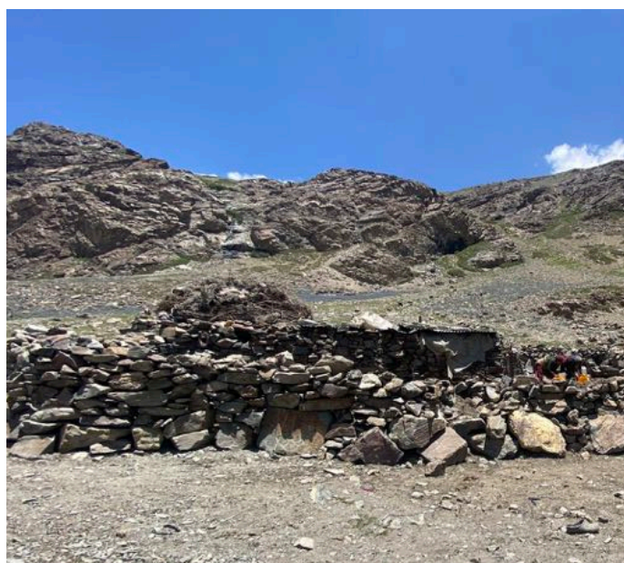
Figure 61 Dry stone masonry walls of the doksa at Abran
