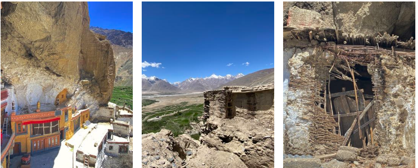
Figure 38 Walls of Phuktal monastery with natural based pigments from locally sourced stone and mud Figure 39 Stone masonry with natural based plaster at Karsha Figure 40 Wattle and daub
