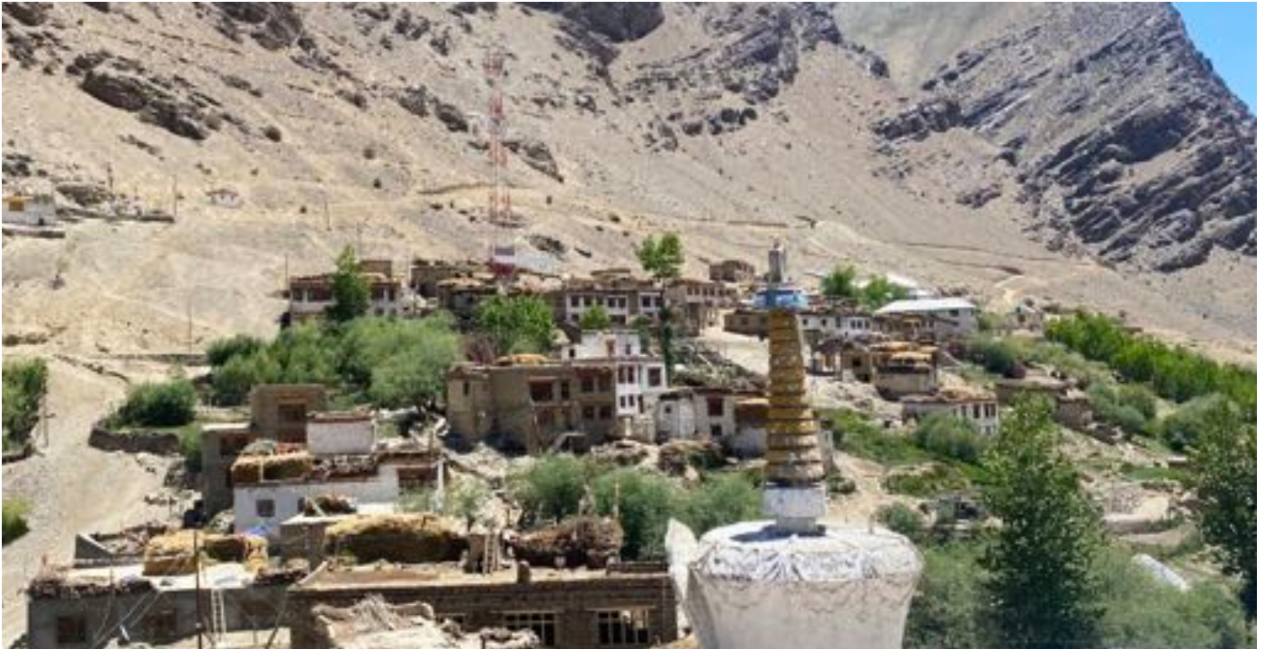
Figure 50 Icher village, the structures are built facing the south/ south-west facing to get maximum exposure of the sun, and thus the maximum percentage of openings are along this facade.
