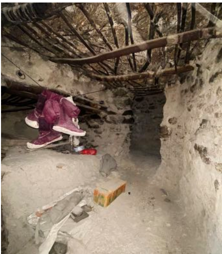
Figure 63 Stone masonry walls with mud based mortar and plaster. The floor is constructed by placing layers of willow sticks, dried shrubs and finished by levelling it with a mud mix
