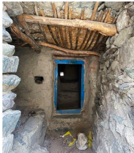
Figure 63 Stone masonry walls with mud based mortar and plaster. The floor is constructed by placing layers of willow sticks, dried shrubs and finished by levelling it with a mud mix
