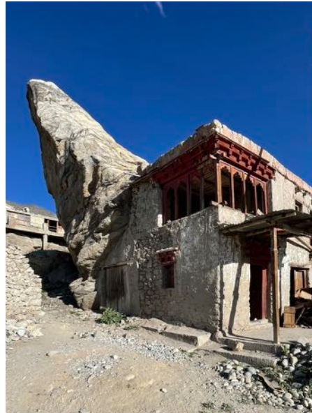
Figure 41 & 42 Construction of structures have complemented and used the natural terrain. Big immovable boulders are accommodated within the structures as seen in Karsha and Padum
