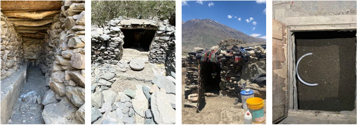
Dry stone masonry wall construction is one of the common process of construction. It is used in the walls of a zing near Lungmi (Figure 34); ranthak at Stongdey (Figure 35) & doksa at Abran (Figure 36). Figure 37 Earthen grain storage shaft at Purne, Zanskar
