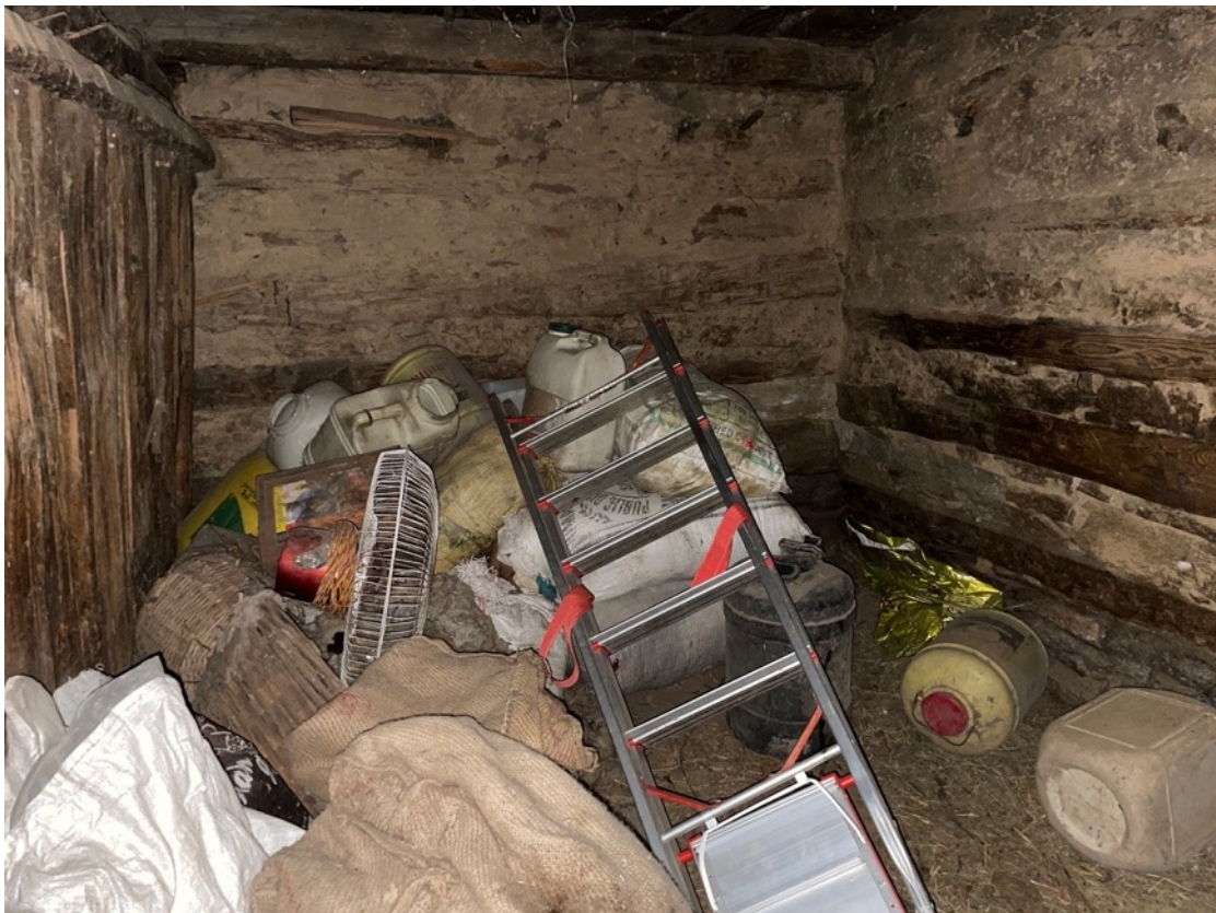
Fig. 18: Unfinished walls of the khudh Source: author
