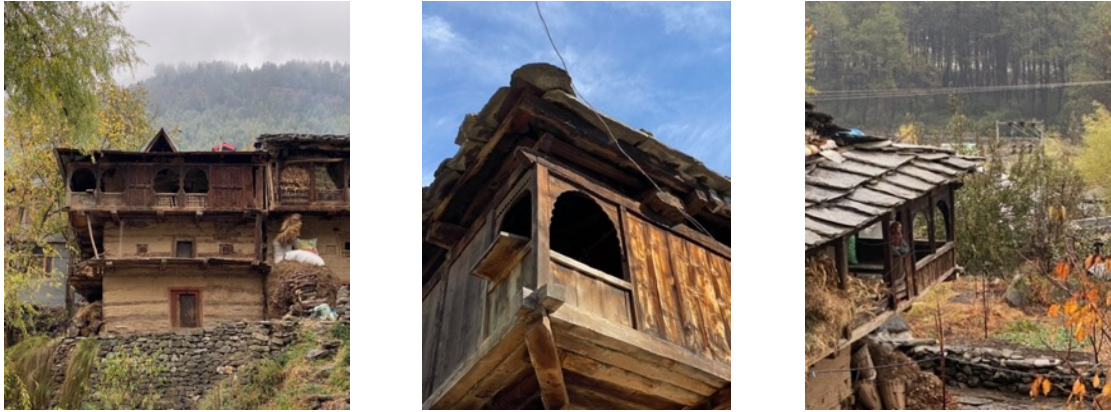
Fig. 10: Traditionally houses in the region were built using stone, timber and slate Source: author
