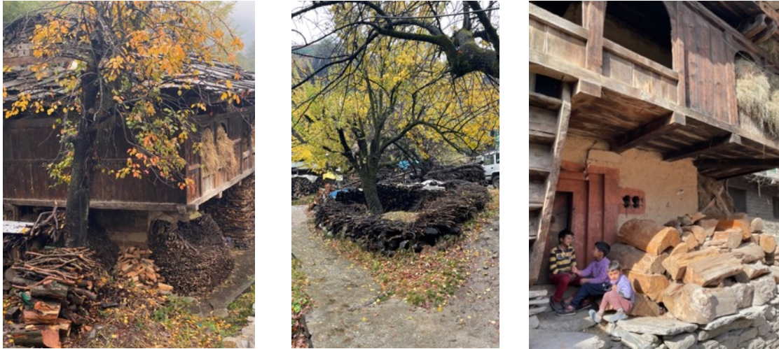
Fig. 15: Variation in firewood stacking in and around the house Source: author
